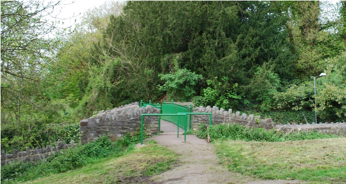
Above: View of existing bridge prior to safety scaffolding
