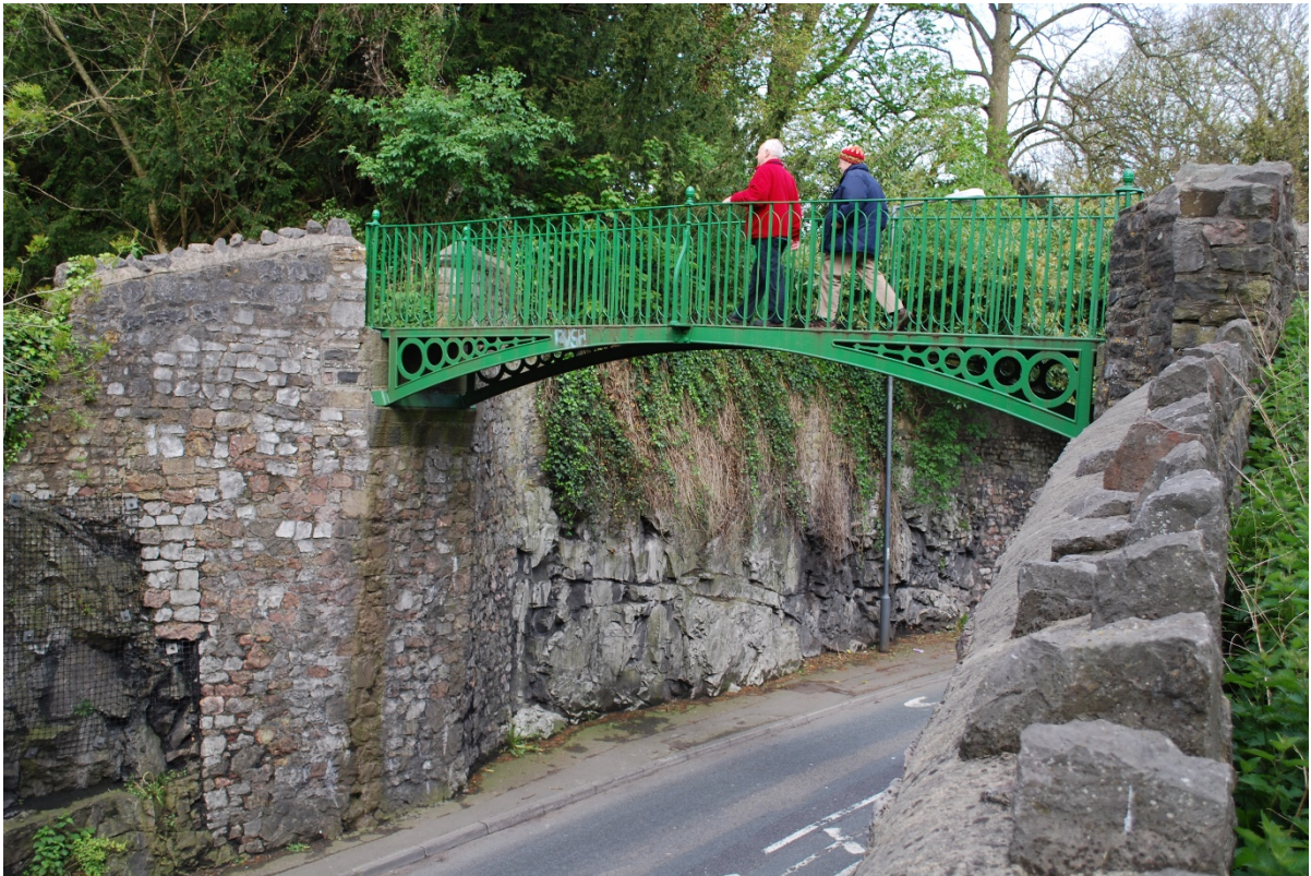
Above: View of existing bridge prior to safety scaffolding
